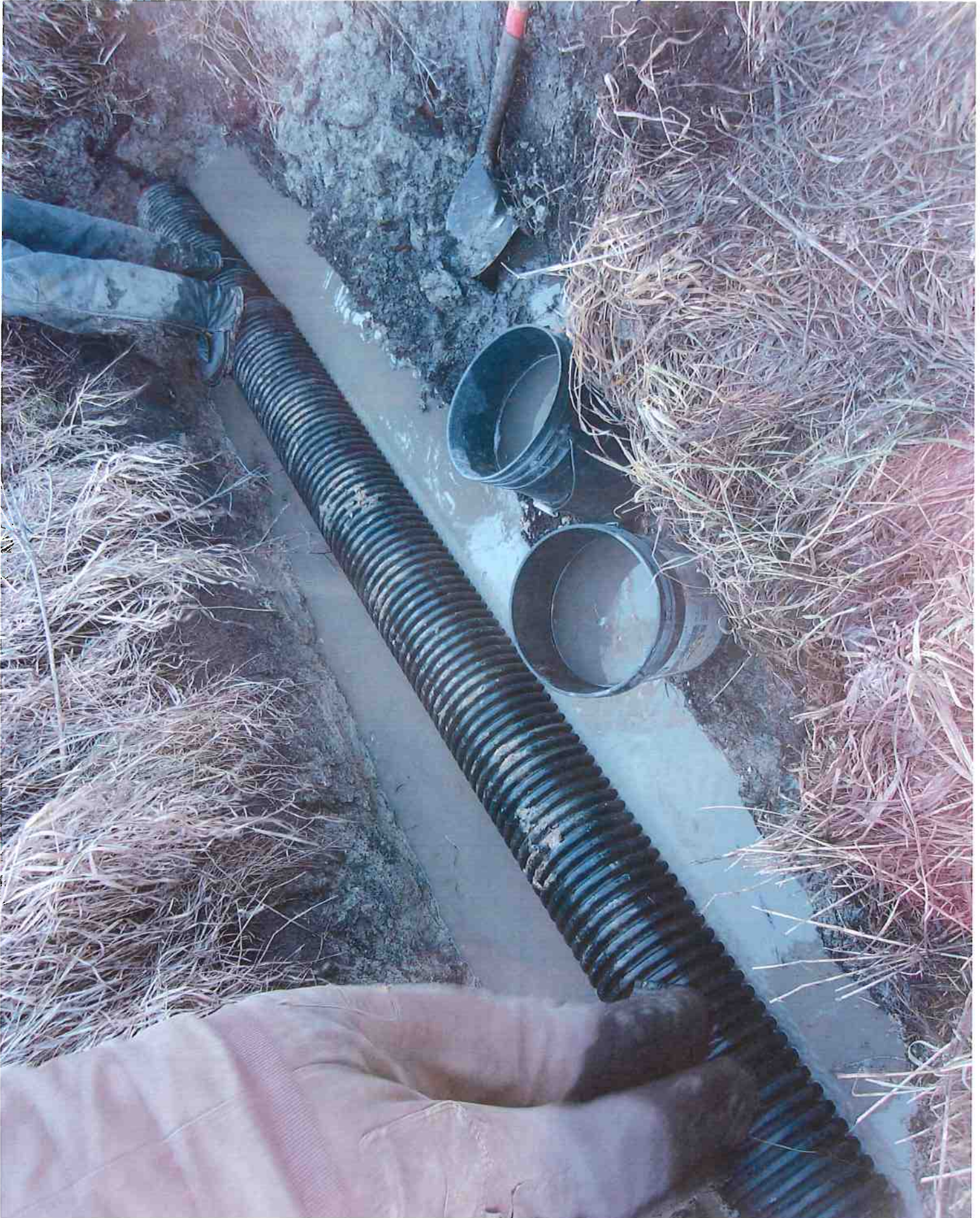
14' of HOPE 10" ON 4" OF BRIDGING ROCK AND HARD CLAY
