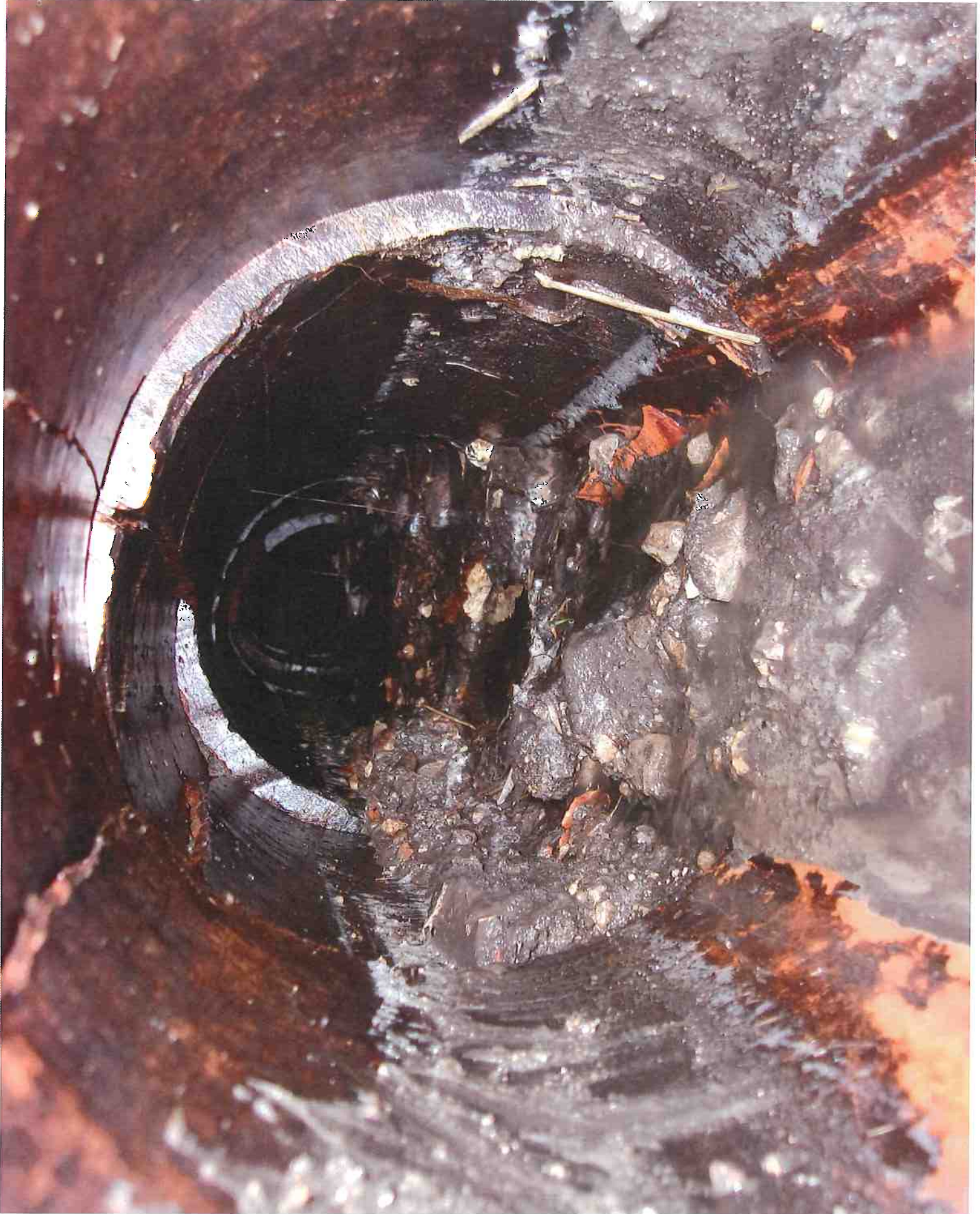
DOWNSTREAM END OF REPAIR
